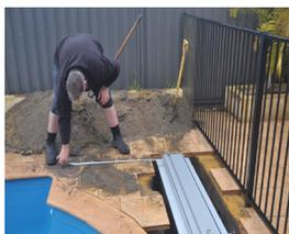
10. Place supplied spacers between lid and front extrusion on the box prior to back filling.
