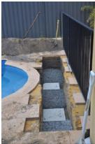
5. Level these slabs so they are approx. 512-515mm below the finished height of paving or concrete. Place spirit level on pool headers and lay across the trench propping the other end up so spirit level is level, using the level measure down to slabs to obtain correct depth of slab, use rubber mallet to tape down to bed slab in.
