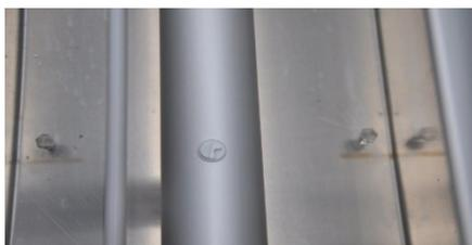
9. Once box is level measure the distance away from pool headers so they are the same either side within a couple of millimetres.
