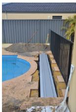
8. With box in the hole and end braces are sitting on concrete slabs level box up to required height via the 4 bolts inside the box, screw all 4 down so they touch the concrete slabs and then every 1 turn gives you approx. 1mm of lift.
