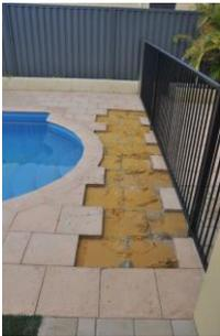
2. Dig trench to minimum of 550mm wide, 555mm deep and at least 300mm past either side of the pools waterline edge. *For example if pool is 4000mm wide dig trench 4600mm long.*
