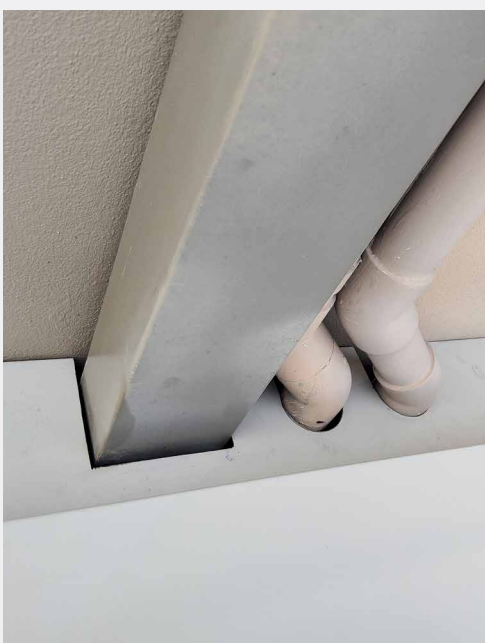
Wall strip has been cut to fit the down pipe and other conduits.
